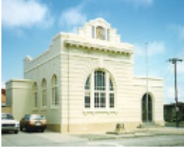
B6498 Former Court House
