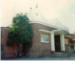
B6471 Old Shire Hall
