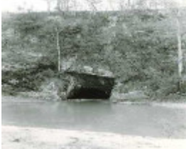
B3121 Pound Bend Tunnel
