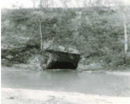
B3121 Pound Bend Tunnel
