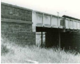
B4022 Railway Bridge
