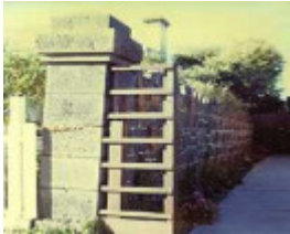
B5595 Wall 10 Twyford Street
