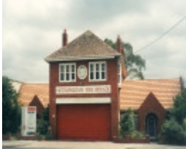
B6894 Fire Station
