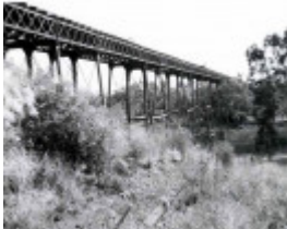
B3741 Railway Viaduct Melton
