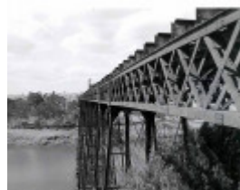
B3741 Railway Viaduct Melton
