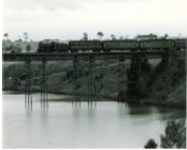
B3741 Viaduct Railway Bridge
