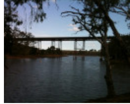
B3741 Melton Viaduct Railway Bridge
