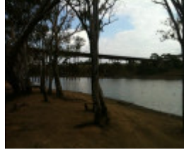
B3741 Melton Viaduct Railway Bridge
