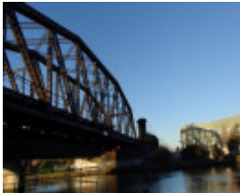
B5745 Rail Bridge over Maribyrnong River
