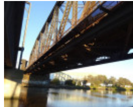
B5745 Rail Bridge over Maribyrnong River substructure
