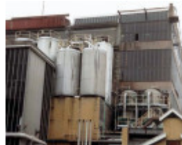
B5089 Main Refinery & New Boiler
