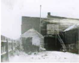
B4197 Old Bakery Building
