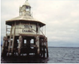
B4357 South Channel Pile Light
