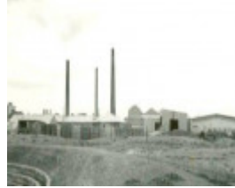
B5546 Frmr Hoffman Brickworks
