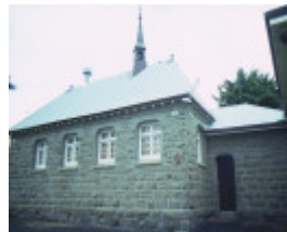
primary school no 2162 grove road lorne side elevation jul1984
