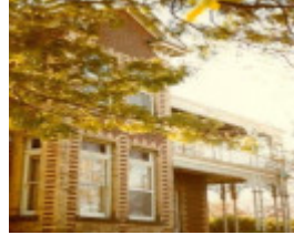
B5527 Frmr Superintendent's House
