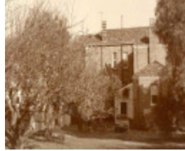
B5527 Frmr Superintendent's House
