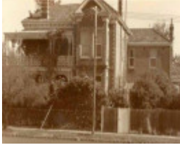
B5527 Frmr Superintendent's House
