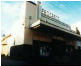
B7008 Progress Hall
