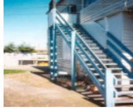
B7110 Outside Stairs
