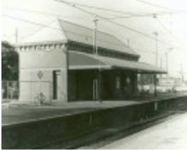
B4933 Moreland Rail Station
