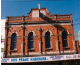
B6707 First Floor Facade H.Bates Building
