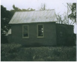
B3144 Uniting Church Former Presbyterian
