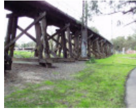
B4173 Eltham Rail Bridge
