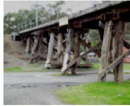
B4173 Eltham Rail Bridge
