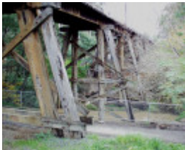
B4173 Eltham Rail Bridge
