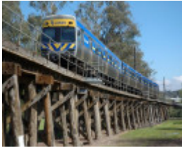
B4173 Eltham Rail Bridge
