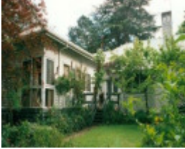
B7141 Bedroom Wing & Main House
