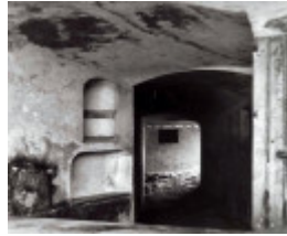
B2165 Corridor Linking Gunposts with Observation Points
