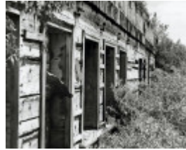
B2165 Former Living Quarters now Stores
