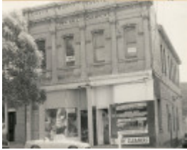
B4232 Town Hall Chambers
