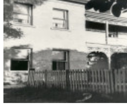
B5208 Holy Trinity Church & Manse 162 Bay St Port Melbourne
