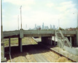
B6228 Centenary Bridge
