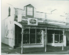
B5218 92-94 Bridge Street
