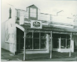
B5218 92-94 Bridge Street
