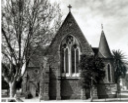
B2154 Holy Trinity Anglican Church Brighton Road Frontage
