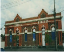
B3938 Former Cable Tram Engine Shed
