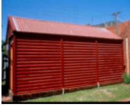
B2240 Portable Iron Houses Complex
