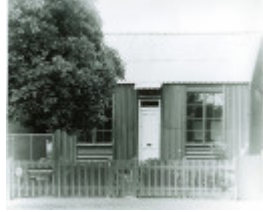
B2240 Portable Iron Houses Complex
