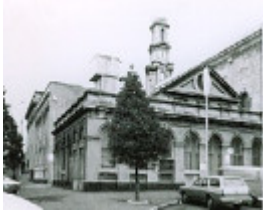
B0577 City Engineer's Office Daly St South Melbourne
