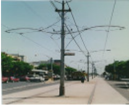
B6438 Ornamental Tram Poles
