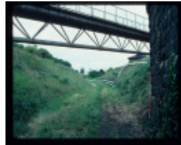
RAILWAY BRIDGE AND CUTTING
