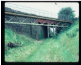
RAILWAY BRIDGE AND CUTTING
