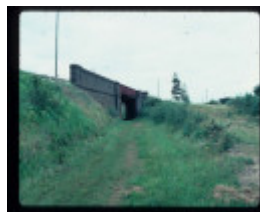
RAILWAY BRIDGE AND CUTTING
