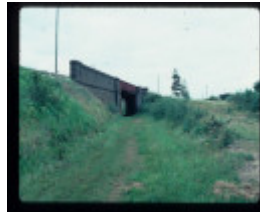
RAILWAY BRIDGE AND CUTTING
