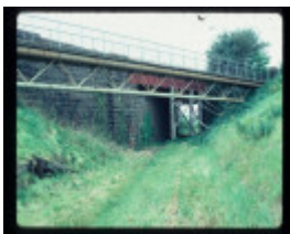
RAILWAY BRIDGE AND CUTTING
