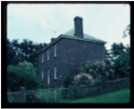
WATTLE HILL HOUSE, WILSONS RD, PORTLAND WEST
