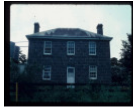
WATTLE HILL HOUSE, WILSONS RD, PORTLAND WEST
