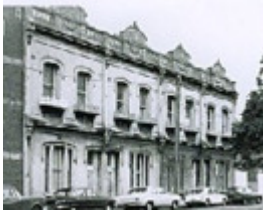
B3987 5-8 Layfield Street
