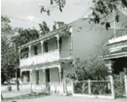
B0216 Park House St South Melbourne
