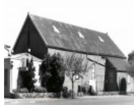
B2645 Cnr Bridge, Prince & Station Streets
