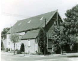
B2645 Cnr Bridge, Prince & Station Streets
