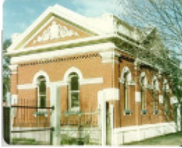
B4602 Gas Valve House
