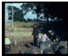
LAKE CONDAH DORMITORY EXCAVATION
