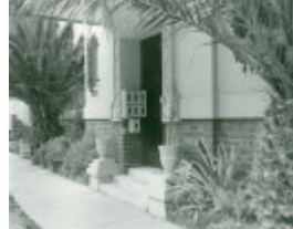
B7083 Belvedere Flats Front Entrance
