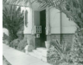
B7083 Belvedere Flats Front Entrance
