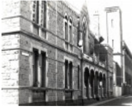
B2437 Court House & Police Station
