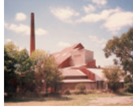
B5992 Box Hill Brickworks
