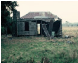
6675 33 Feature 1 South wall of hut
