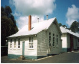
B6691 Primary School No 2838 & Sloyd Room
