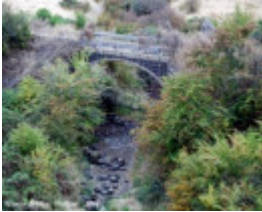
B6074 Bridge Inn Road Bridge
