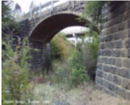
B6074 Bridge Inn Road Bridge
