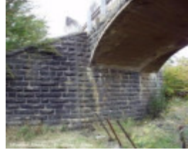
B6074 Bridge Inn Road Bridge
