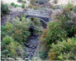
B6074 Bridge Inn Road Bridge
