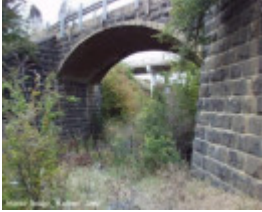
B6074 Bridge Inn Road Bridge
