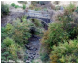
B6074 Bridge Inn Road Bridge
