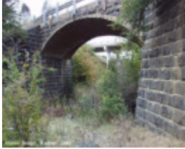
B6074 Bridge Inn Road Bridge
