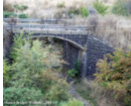
B6074 Bridge Inn Road Bridge
