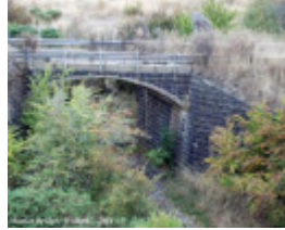
B6074 Bridge Inn Road Bridge
