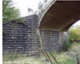
B6074 Bridge Inn Road Bridge
