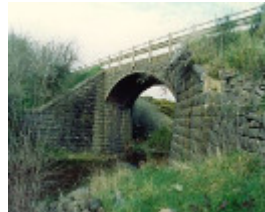
B6074 Bridge Inn Road Bridge
