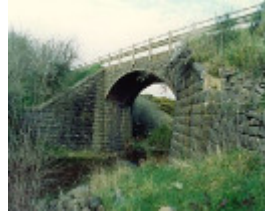
B6074 Bridge Inn Road Bridge
