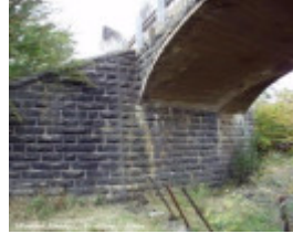
B6074 Bridge Inn Road Bridge
