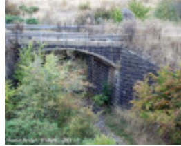
B6074 Bridge Inn Road Bridge
