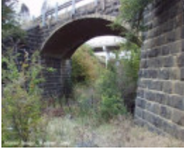
B6074 Bridge Inn Road Bridge
