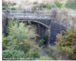
B6074 Bridge Inn Road Bridge
