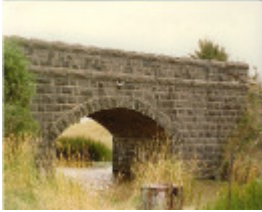
B1577 Bluestone Bridge
