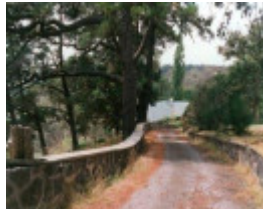
B7166 Farm Vigano Driveway
