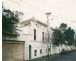
B0229 Tintern House Facade
