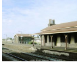
B2285 Rail Station
