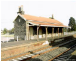
B2285 Rail Station
