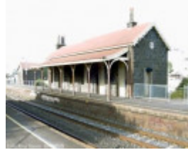
B2285 Rail Station
