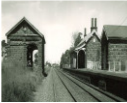
B2285 Railway Station & Goods Shed
