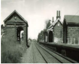
B2285 Railway Station & Goods Shed
