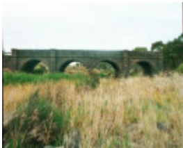
B2055 Rothwell Bridge
