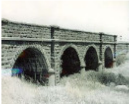
B2055 Rothwell Bridge
