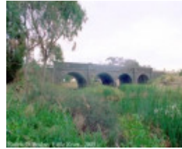
B2055 Rothwell Bridge
