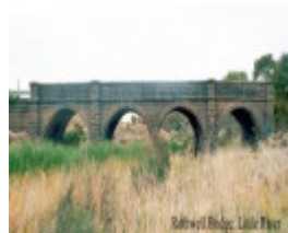
B2055 Rothwell Bridge
