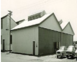
B4309 Building No 210
